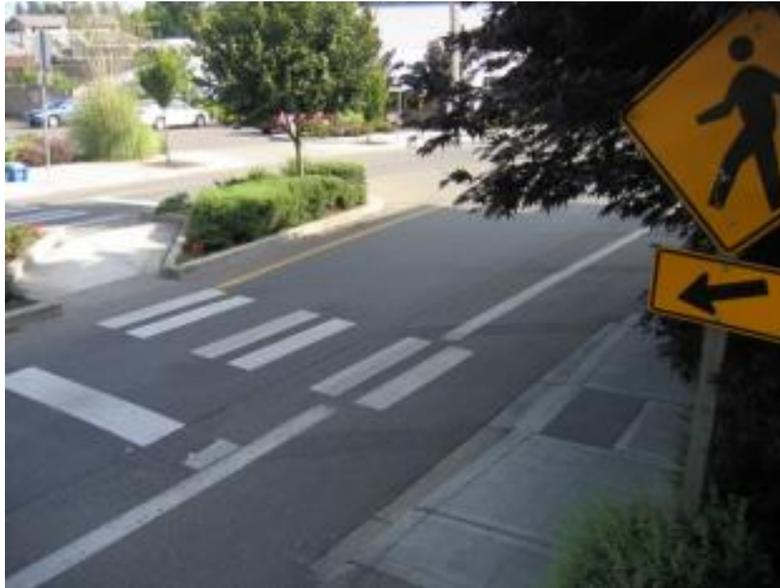
**Figure 19. Marked crosswalk at a midblock location.**
