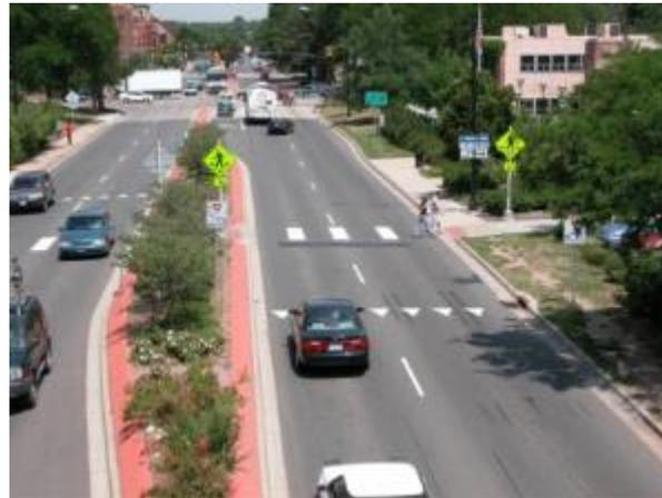
**Figure 8.** The white triangle pavement markings shown here represent the advance yield line. Some states use a solid white line, as shown in Figure 9.
